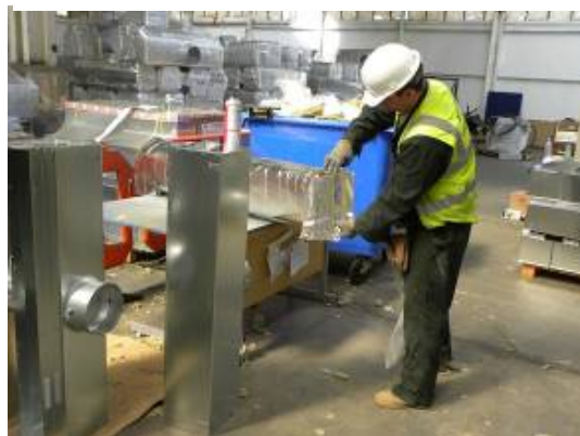
Figure 7 A workstation at the LCCC used for lagging air-conditioning units prior to delivery to site
